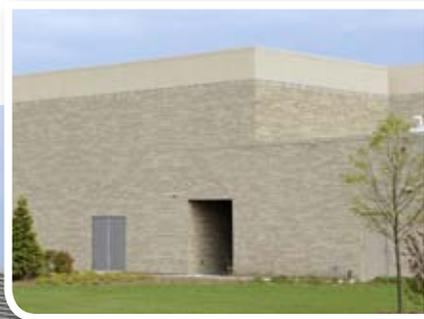
*Harmonize the horizontal line of the brick façade with continuous blade design.*
