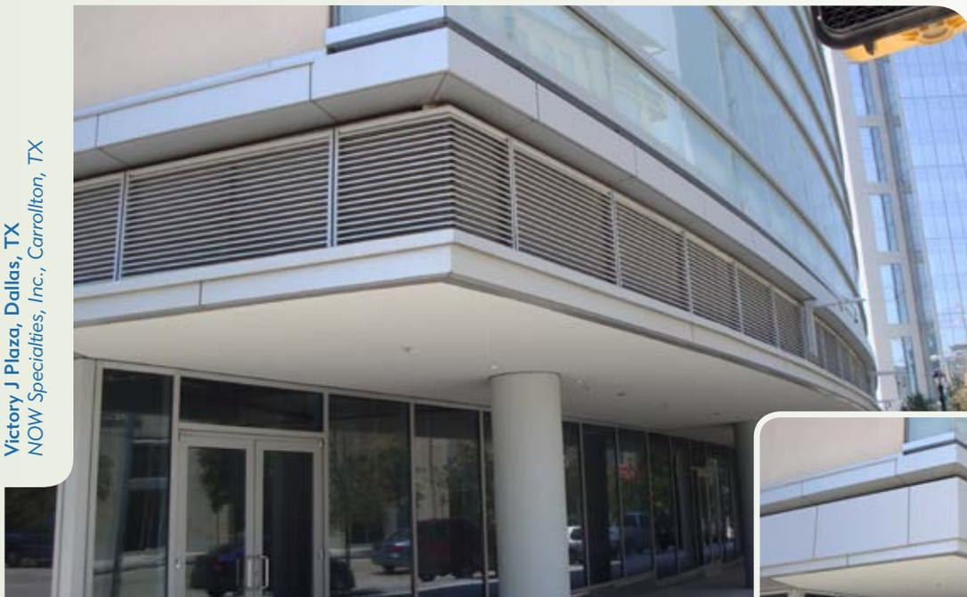
*Complement vertical lines in panels.* Ruskin's EME520DD multi-section louvers with visible mullions match the panel break lines for a consistent appearance.
