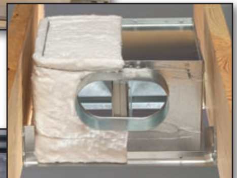
Insulated Plenum Wood Joist
