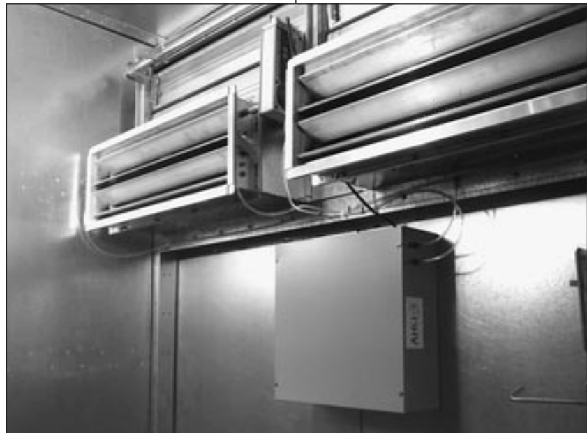
Compliance with ventilation standards should not be costly. The ability of Ruskin's IAQ40 damper to fit into a standard AHU design saved in cost and delivery lead time.
