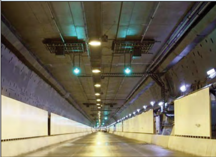
Above: Ruskin model TFD80 (3000mm x 2000mm) built for the Clem Jones Tunnel Project in Brisbane QLD, Australia. Below: TFD80 dampers are installed in the Clem Jones Tunnel ceiling for Emergency Smoke Extraction.
